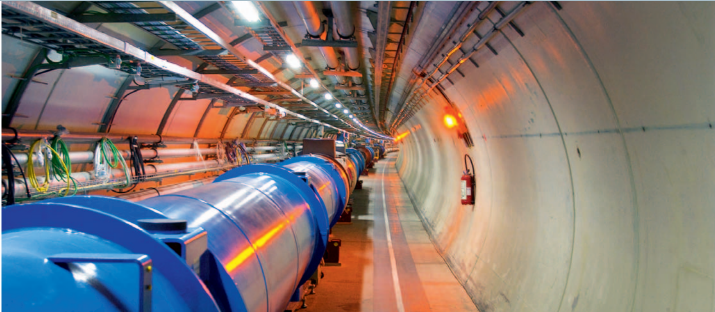
3 In the particle accelerator tunnel
